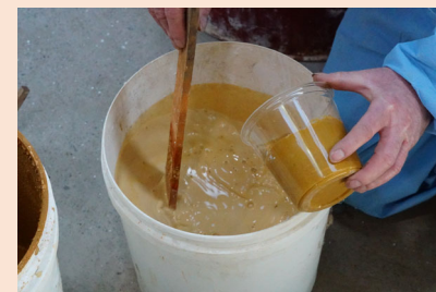
Mixing limewash at the Works Depot
