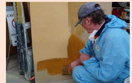
Colour matching limewash at the Works Depot
