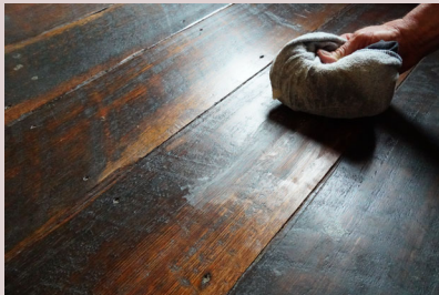
Applying beeswax polish to timber flooring
