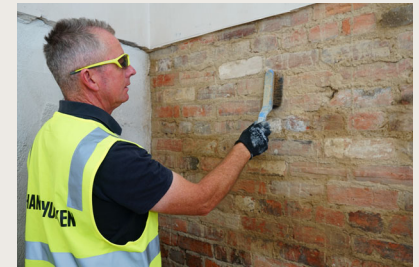
Cleaning excess dust from the surface
