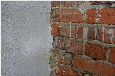
Determining the extent of salt damp
