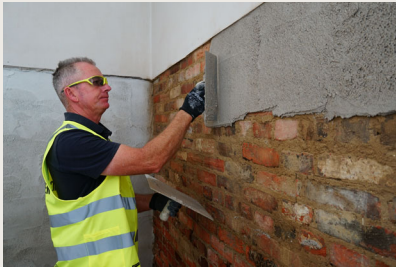
Applying sacrificial lime render to brickwork
