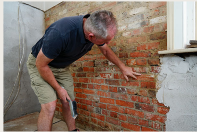
Determining the extent of salt damp
