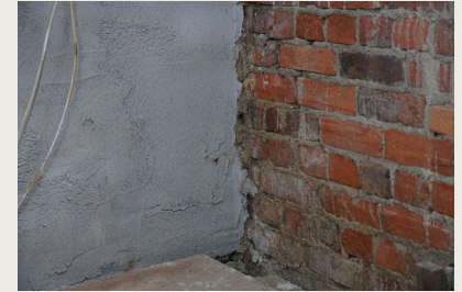
Evidence of salt damp
