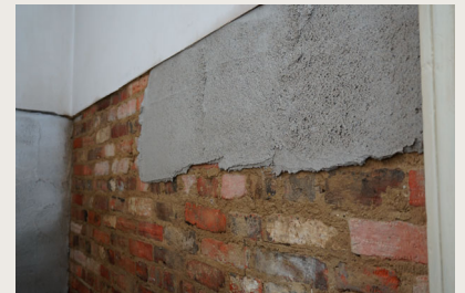
Applying sacrificial lime render
