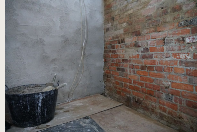
Evidence of salt damp
