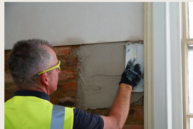
Applying sacrificial lime render
