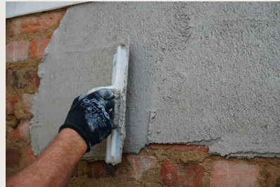
Applying sacrificial lime render to brickwork
