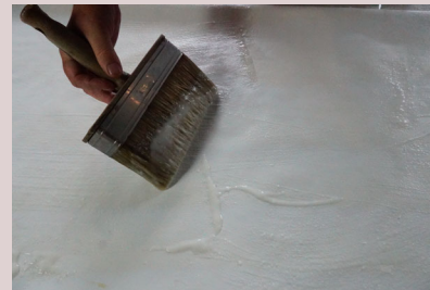
Applying glue and folding
