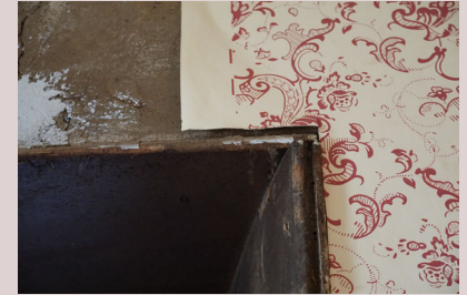
Rough plaster and uneven joinery
