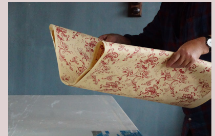
Applying glue and folding
