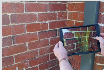
Determining extent of mortar deterioration
