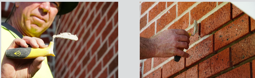
Repointing lime mortar joints in brickwork
