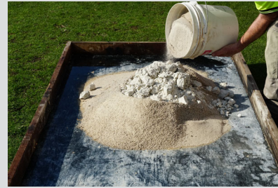
Preparing sand-slaked lime mortar
