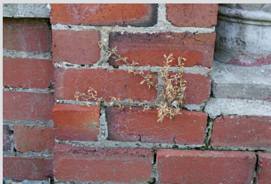
Determining extent of mortar deterioration
