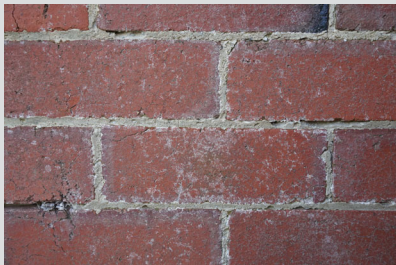
Deteriorated mortar joints
