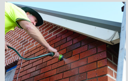
Preparing joints for repointing
