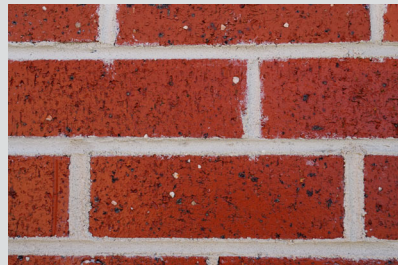
Repointed lime mortar joints
