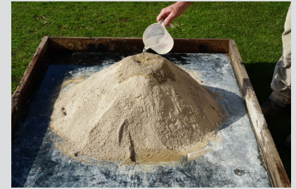
Preparing sand-slaked lime mortar
