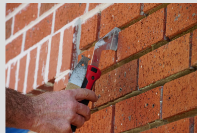
Preparing joints for repointing
