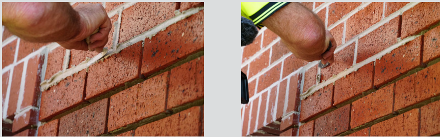
Repointing lime mortar joints
