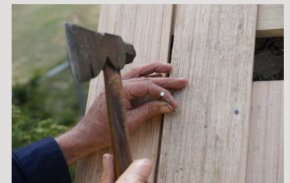
Fixing dry shingles
