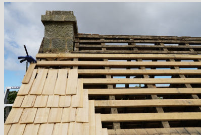
Replacing a timber shingle roof
