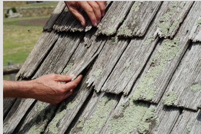
Determining length, width and thickness for shingles
