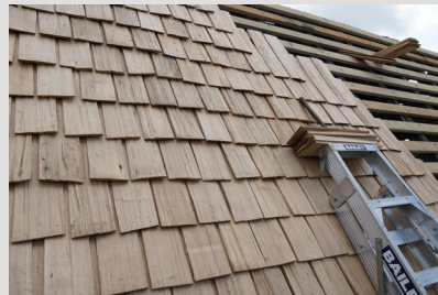
Fixing shingles to battens
