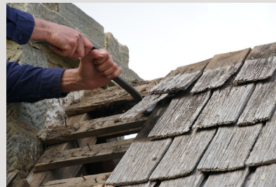
Removing damaged shingles and battens
