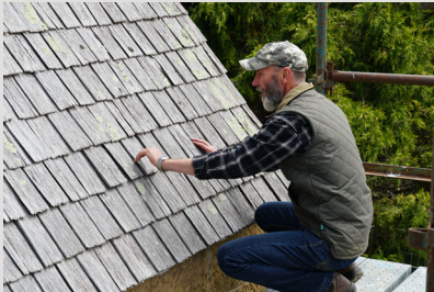
Determining length, width and thickness for shingles
