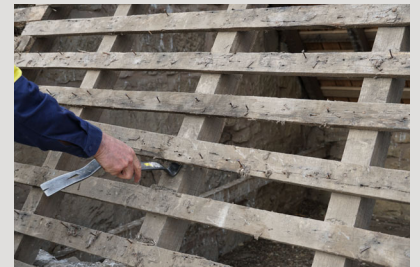
Removing damaged shingles and battens
