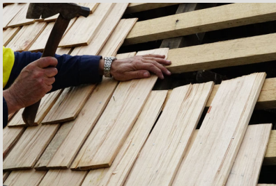
Fixing shingles to battens
