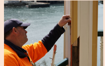
Checking condition of timber behind skirting
