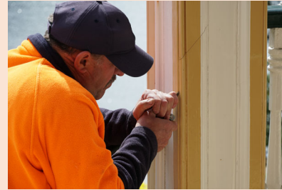
Removing damaged skirting
