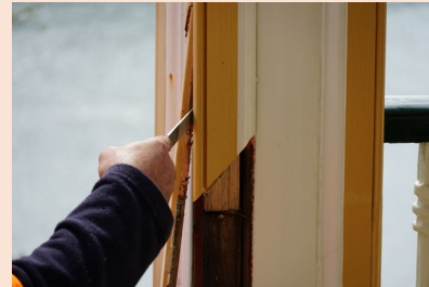
Checking condition of timber behind skirting
