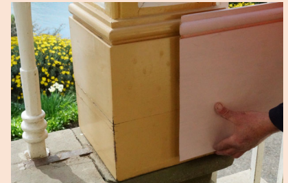
Matching moulding at the Commandant's House
