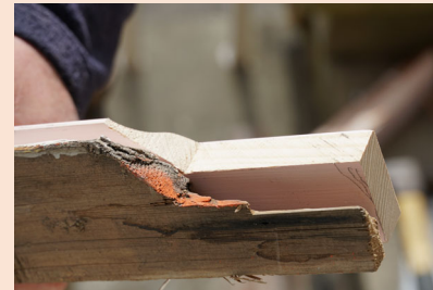
Matching moulding at the Commandant's House
