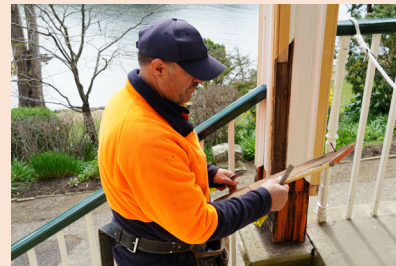
Inspecting and repairing damaged skirting
