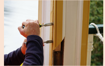
Removing damaged skirting
